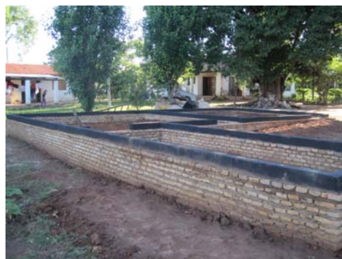
Foundations for Work >>
